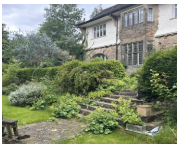
A Characteristic Arts & Crafts treatment using natural materials: the lower storey is faced in local stone from the Bell Hagg Quarry contrasting with the roughcast walls above. The roof is constructed of Brighthouse stone slates
