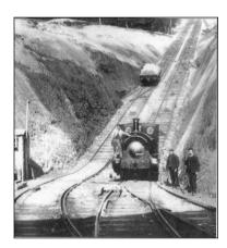
At the Bole Hill quarry, face stone was loaded into rail cars and winched down the 1 in 3 railway incline shown in the photo above and which it is still possible to see, although much overgrown. From the sidings at Grindleford station, stone was assembled into trainloads to be hauled along the main line to further sidings just beyond Bamford station. In order to create the link to the dam sites in the Upper Derwent
